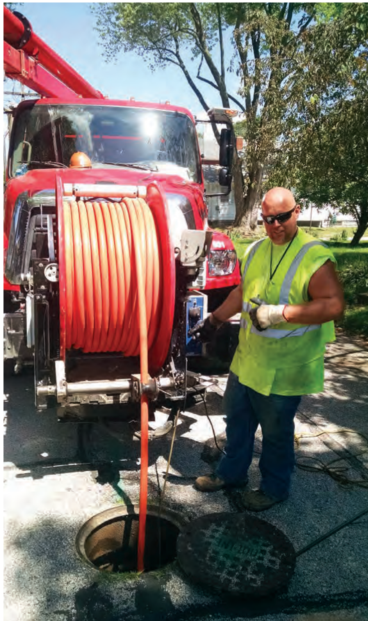
AFSCME Local 1132 member James Gordon jetting a sewer line in Moline.
